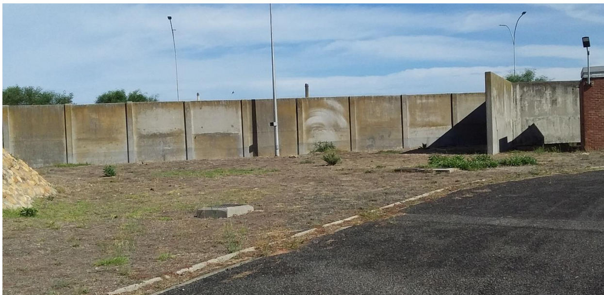
Diagram 3: setup of SFF Milnerton boundary wall, approx. 4 meters high.
